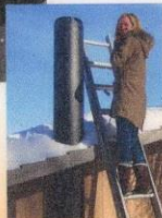
A Teton Raptor Center vent screen. The Poo-Poo Project's goal is to prevent wildlife entrapment within vent pipes without compromising ventilation by installing these screens across the U.S. Right: A TRC volunteer installs a vent screen on a vault toilet in Jackson, Wyoming.
